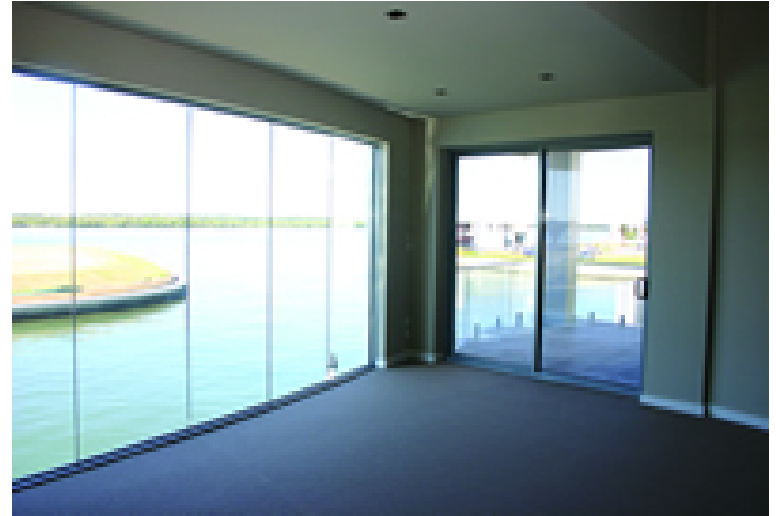
Wall of fixed lites and sliding door
